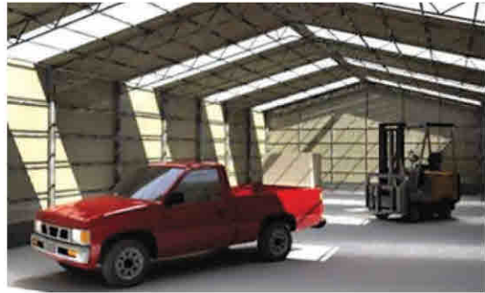
Clear skylight panels can create a harsh indoor lighting environment, with glaring sunlight in some areas and stark shadows in others.
